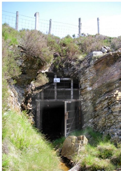
Figure 659: Adit entrance to Prince Edward mine.
