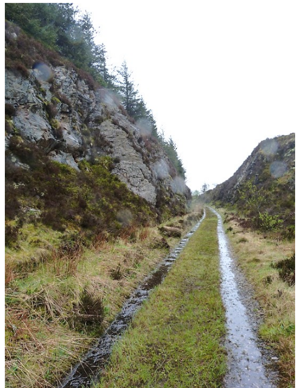
Figure 661: Cutting on the disused railway through Cwm Prysor.
