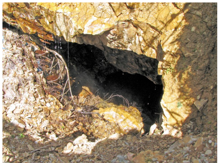
Figure 644: Collapsed entrance to Roberts' level.
