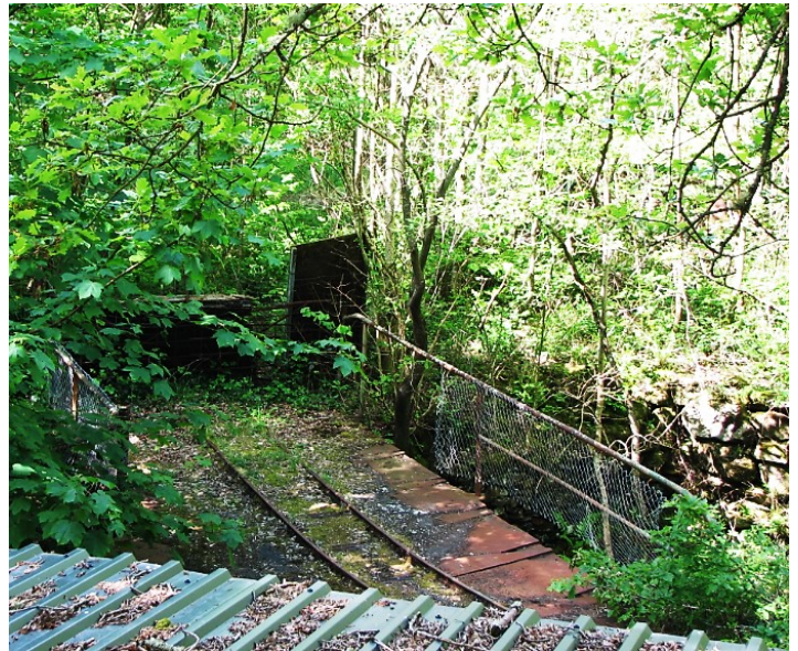
Figure 651: Tramway bridge at the mouth of the Llechfraith adit.
